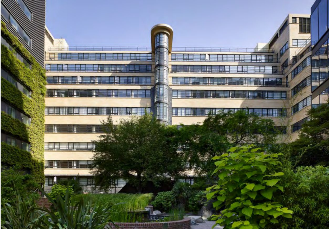
Above: View looking north from Portsoken Street Garden.
