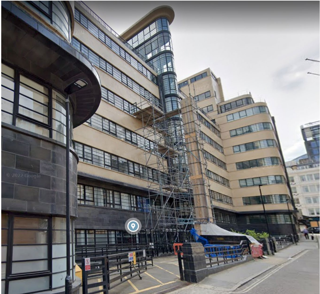
Above: View looking south-west from Haydon Street.
